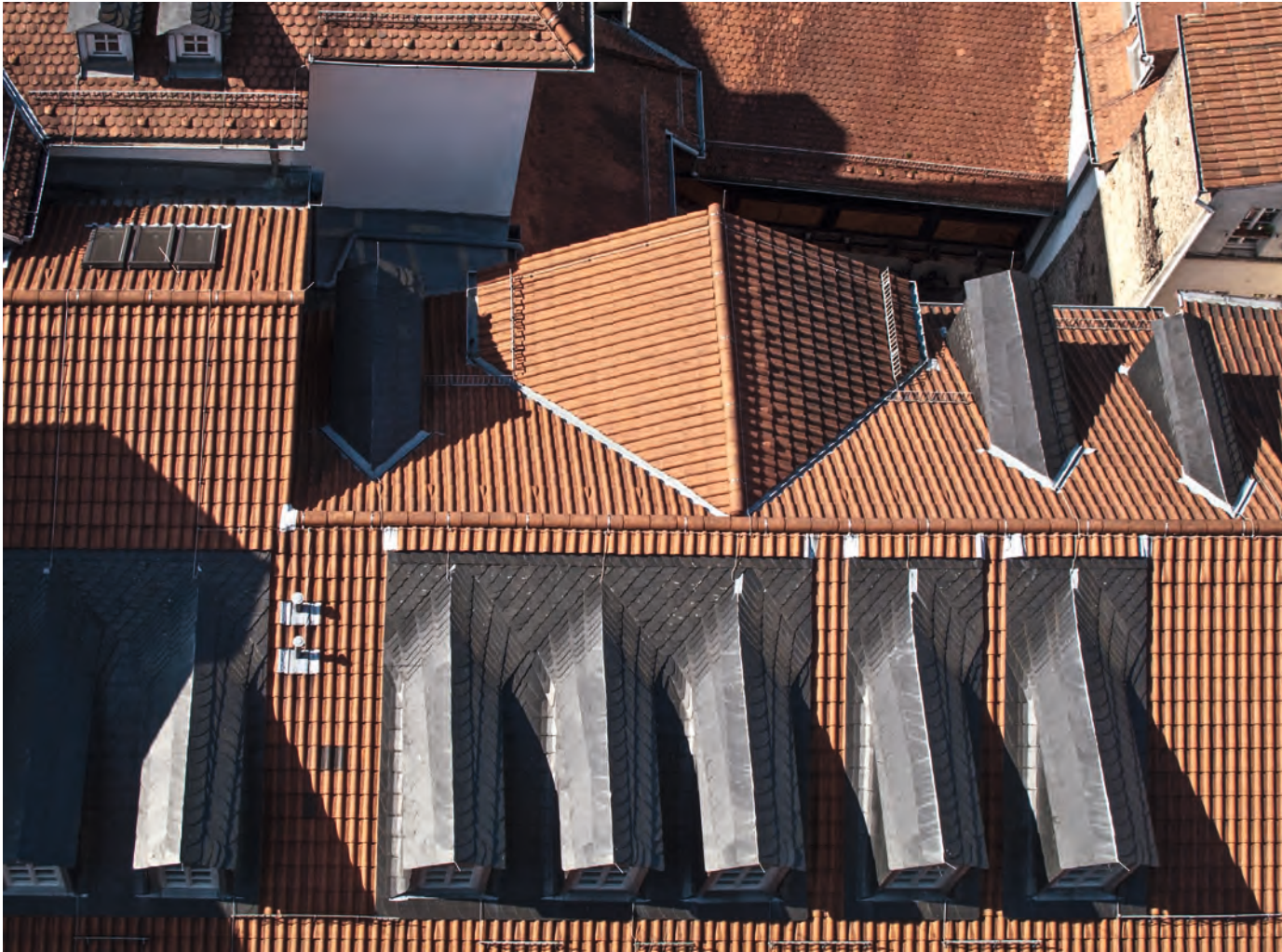
◀ Figure 8-4: Rooftops, Heidelberg In order to take this photograph, I had to hold my camera as far out from the thick tower wall as possible, making it impossible to see the composition before I pressed the shutter button. After several attempts, I was able to square up the image as I wanted, highlighting the abstract geometry of the rooftops below me.
